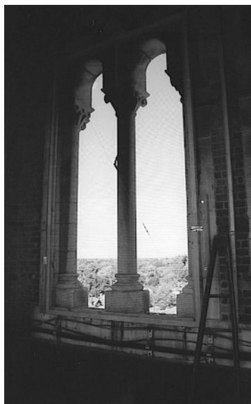
Black nylon mesh screening in bellchamber opening. Once installed, it is virtually invisible.
